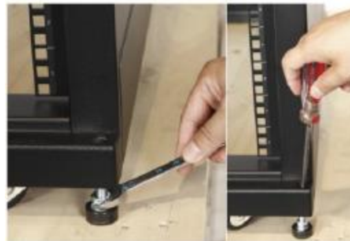
Leveling feet for site leveling
