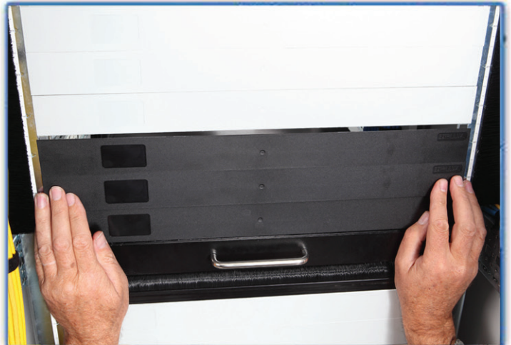
Place the panel in position, aligning the clips with the 19" mounting holes and push into place.
